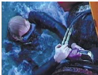
4-XLCT on dredger suction pipe
